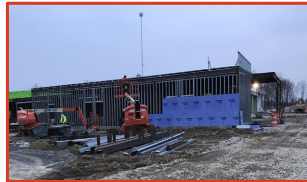
Picture 2: Sheathing Installation in Admin Area
