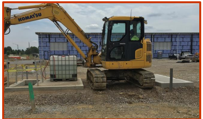
Picture 3: Concrete pads in the courtyard for the transformer and generator
