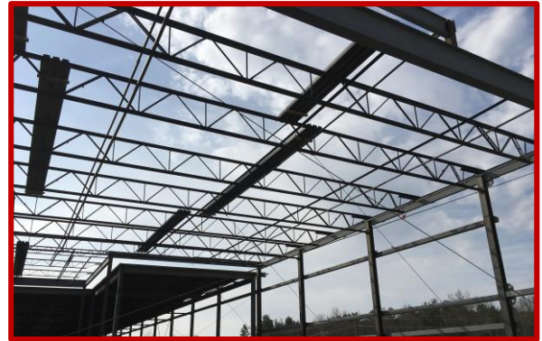
Picture 1: Structural steel joists above Student Dining awaiting metal decking
