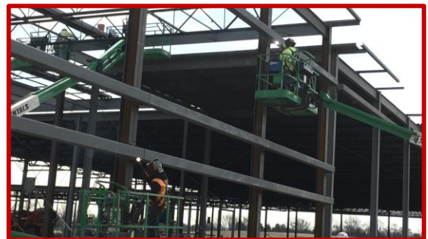
Picture 3: Welding of hollow steel tubes over the doors and windows in Student Dining
