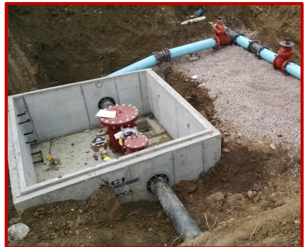
Picture 2: Installation of underground water meter vault
