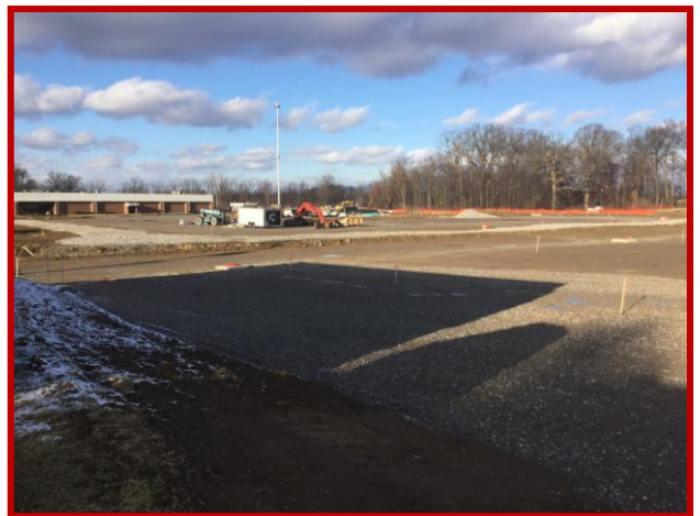
Picture 3: Current view of site ready for foundations
