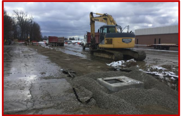
Picture 1: Storm and sanitary line installation ongoing
