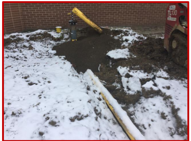
Picture 2: Gas line into the building ready for backfill
