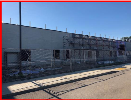
Picture 2: Exterior Masonry at the East Admin Area
