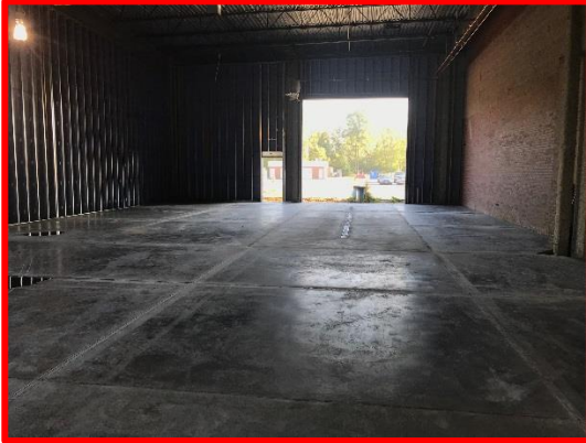
Picture 1: Slab on Grade Placement in Fire Service Tech
