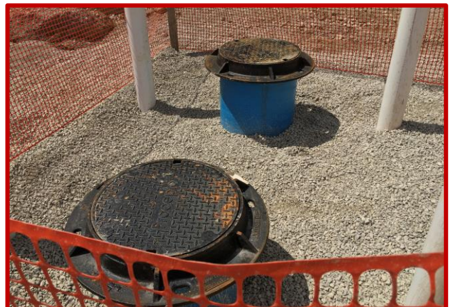
Picture 3: Grease and oil interceptors backfilled in the courtyard
