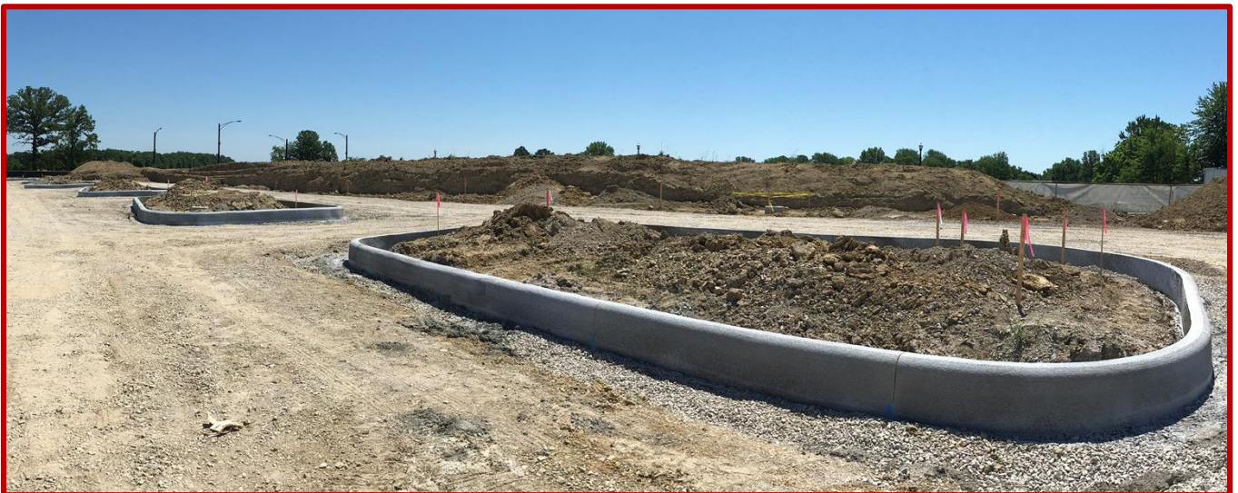
Picture 5: Curing curbed concrete islands in the South parking lot
