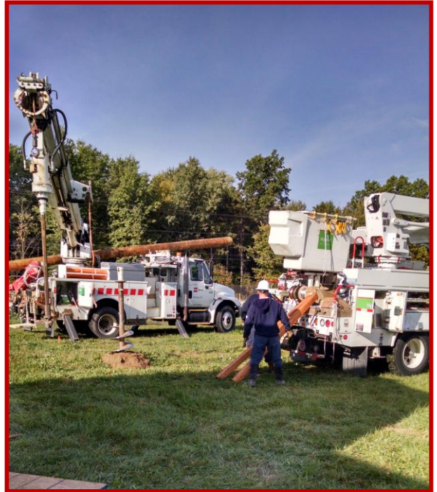
Picture 1: AEP on site setting temporary power poles
