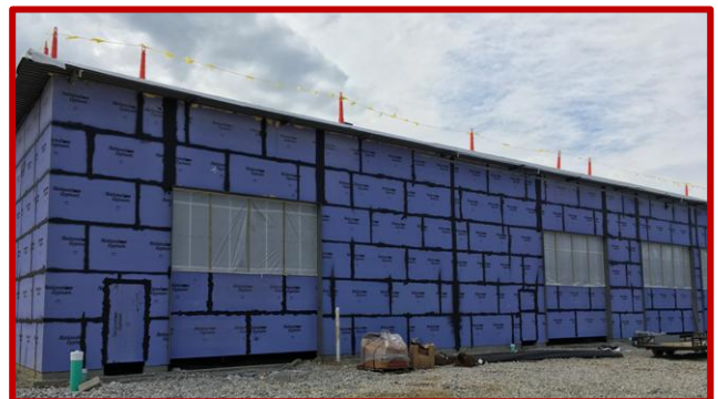
Picture 3: Temporary enclosures at the overhead doors in Area A
