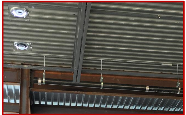
Picture 1: Installation of roof drains in progress in Area D
