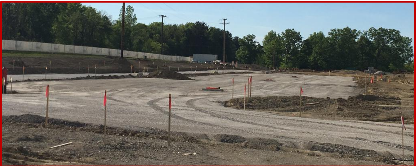
Picture 5: Gravel base at the South West parking lot along the West side of Areas B and C
