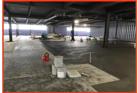
Picture 1: Slab on Grade in Culinary Arts
