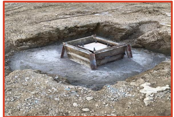
Picture 2: Concrete foundation at Building tie-in
