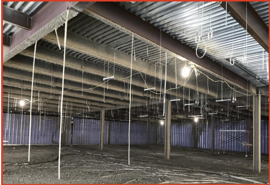
Picture 3: Fireproofing of 2 nd Floor Mezzanine
