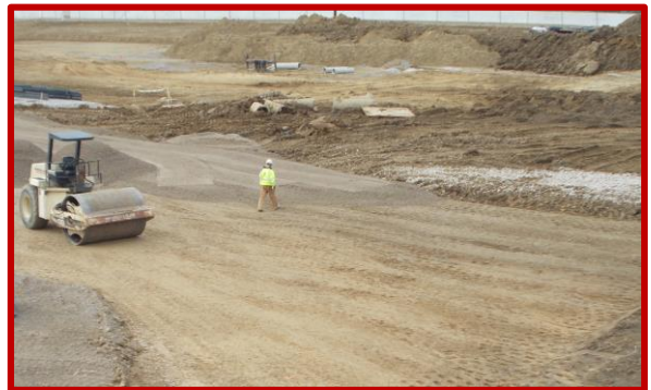
Picture 2: Progress on the building pad in Area D
