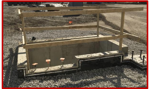
Picture 1: The elevator pit installed in Area D
