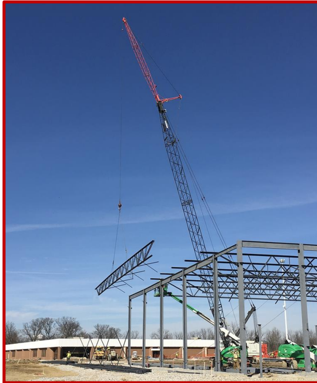
Picture 4: Steel trusses being lifted into place in Area B
