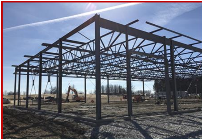
Picture 5: Progress in Area A; columns beams, and trusses
