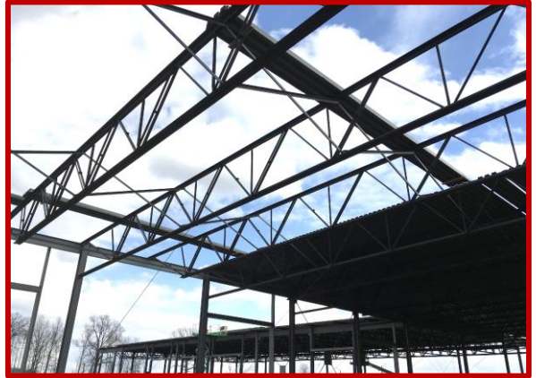
Picture 1: Progress of metal decking installation in Area C
