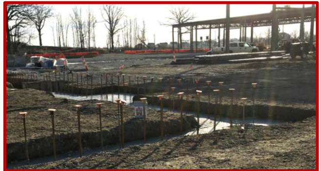
Picture 2: Concrete foundation for the firewall between Areas C & D
