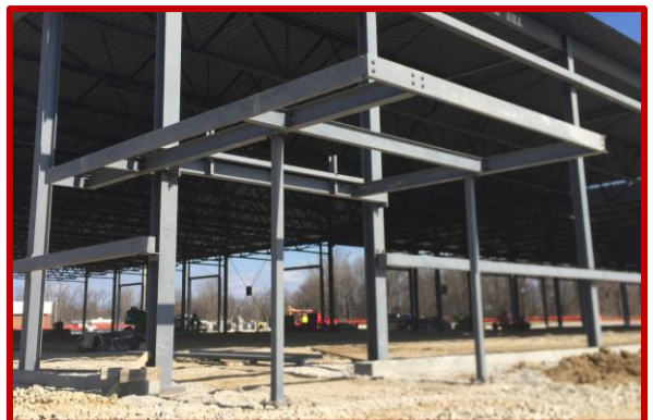
Picture 3: Steel in place for the entry vestibule in Area B
