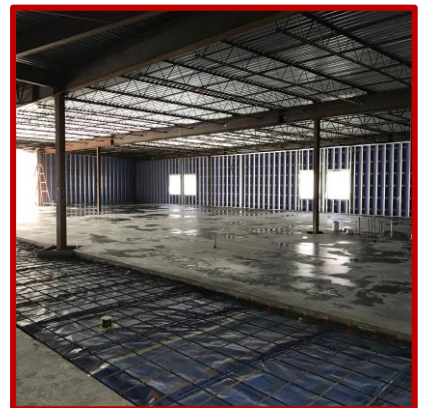
Picture 3: Slab on Grade pour in new Admin Area
