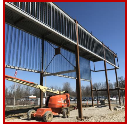
Picture 1: Light Gauge Metal Framing at Connector
