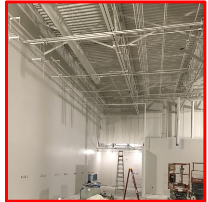
Picture 2: Progress in Welding Lab
