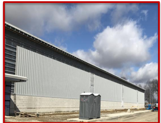
Picture 2: Wall Metal Panels along the South Elevation
