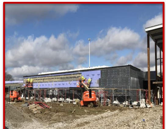
Picture 3: Exterior Insulation of Early Childhood Development Area
