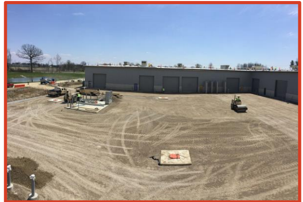
Picture 1: Courtyard Preparation for Asphalt Paving
