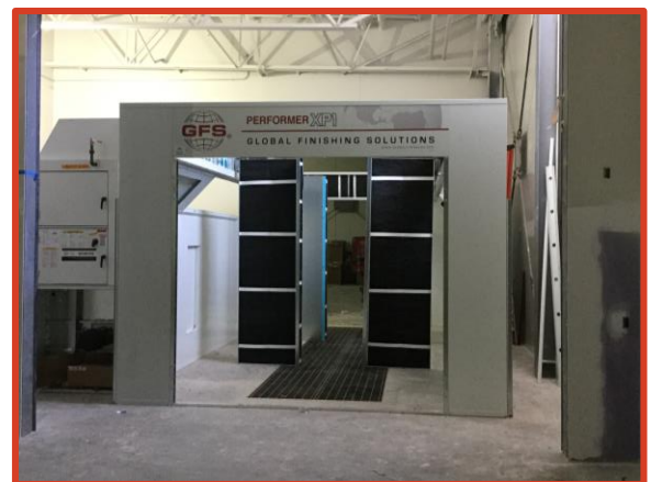
Picture 3: Progress in Auto Collision/Power Sports & Diesel Paint Booth
