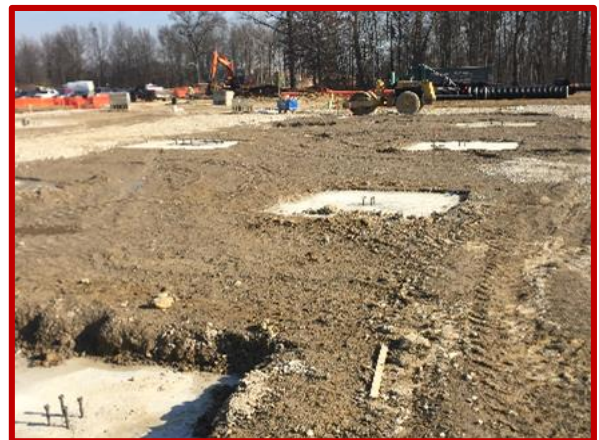
Picture 3: Column footers with anchor bolts set in Area E
