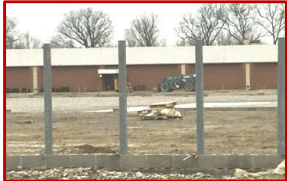
Picture 1: Hollow structural steel in place for windows in Area A
