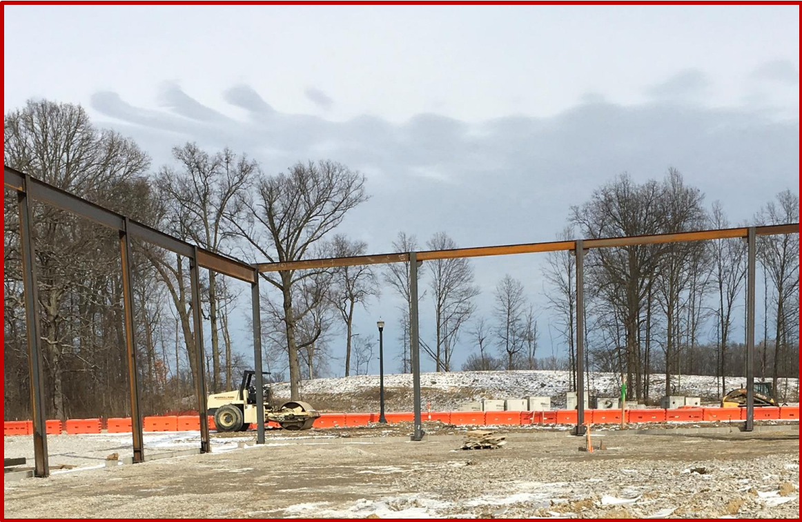
Picture 4: Structural steel erection progressing in Area A
