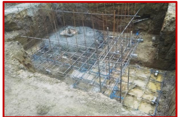
Picture 2: Concrete placement beginning in the elevator pit in Area D
