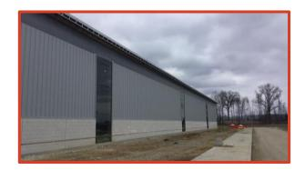
**Picture 3:** Metal Panels and Dynamic Glazing in South Elevation
