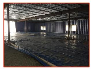
**Picture 1:** Prep for Slab on Grade Pour in new Admin Area
