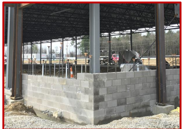
Picture 3: Progress of the masonry firewall and in-wall electrical rough-in
