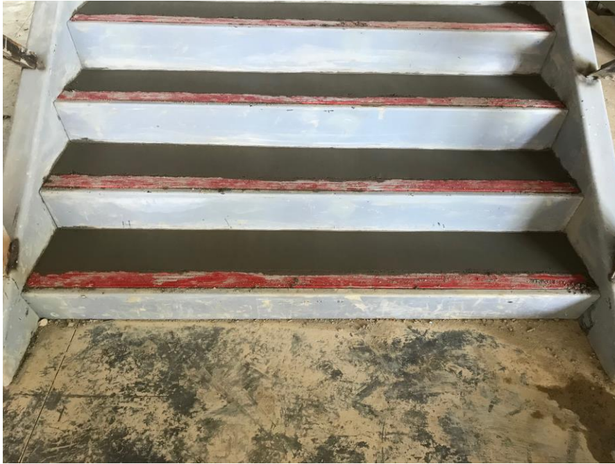
Picture 6: Stair Riser pour in the Connector
