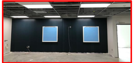
Picture 2: Installation of Markerboards in the Shared Classroom between Power Lines Lab and Construction Tech
