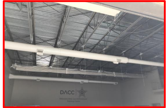
Picture 1: Ceiling Demolition in the Law Enforcement Multi-Purpose Room
