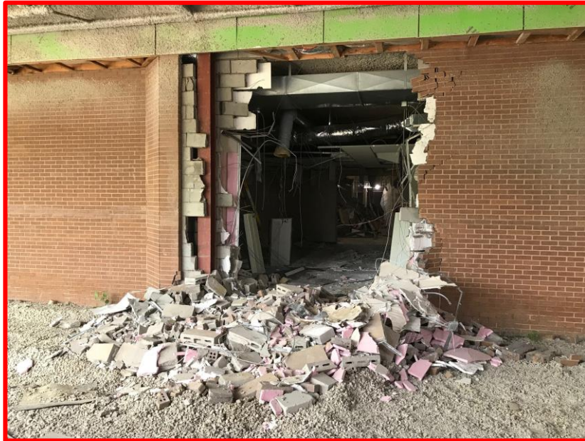
Picture 4: Wall Demolition at New Entrance to Learning Commons
