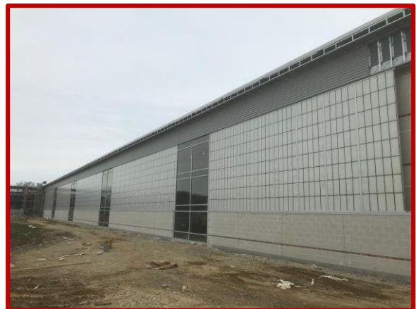
Picture 3: Progress on West Elevation
