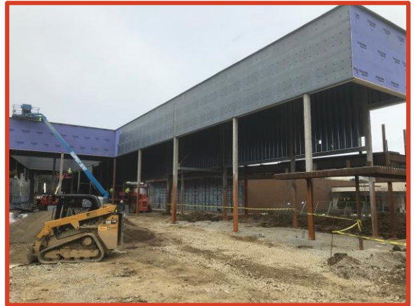
Picture 1: Drywall and Insulation Progress in Connector
