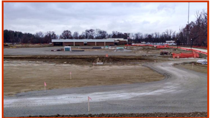
Picture 2: Current progress along the building pad
