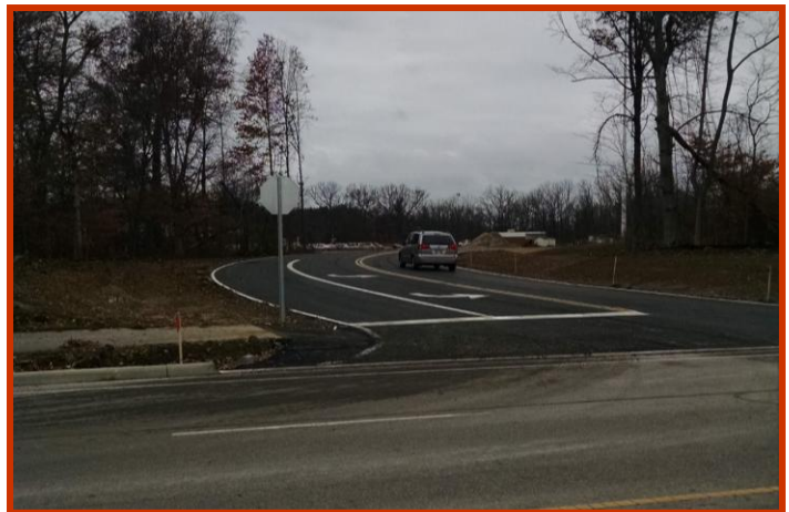
Picture 3: New access road for students and staff
