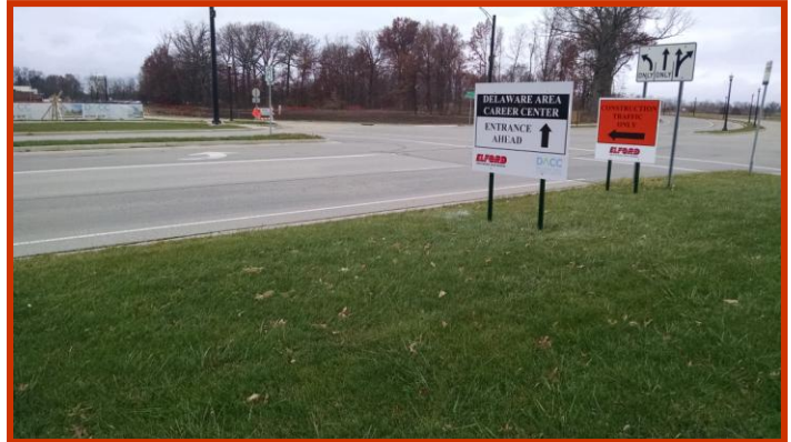
Picture 1: Installation of temporary traffic signage
