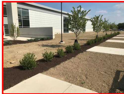
Picture 6: Trees and Shrubs on the West Side of the Building
