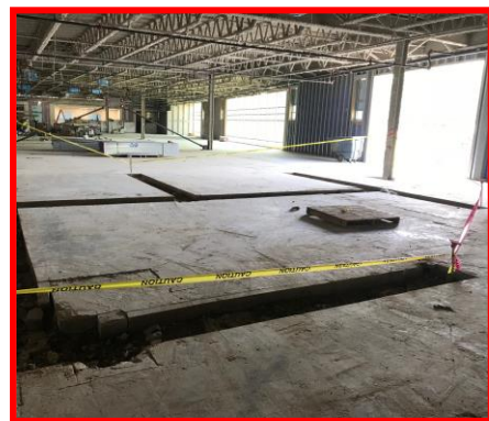
Picture 5: Trenching for Underground Electrical in Area H
