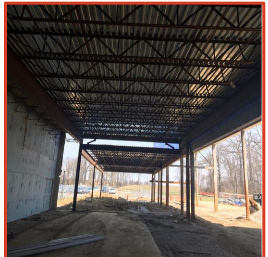
Picture 3: Decking Installed in Connector Area
