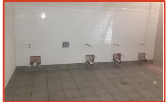
Picture 1: Ceramic Tile in Group Restroom
