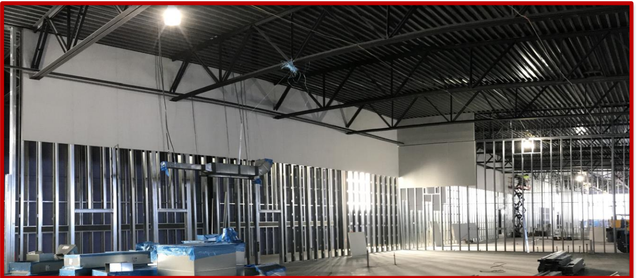
Picture 5: Drywall Top out in Area A
