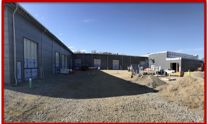
Picture 1: Exterior Insulation in Courtyard Areas
