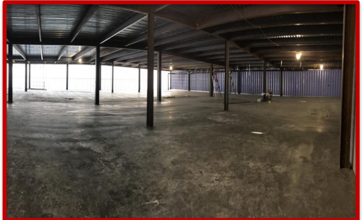
Picture 2: Mezzanine Slab on Deck
