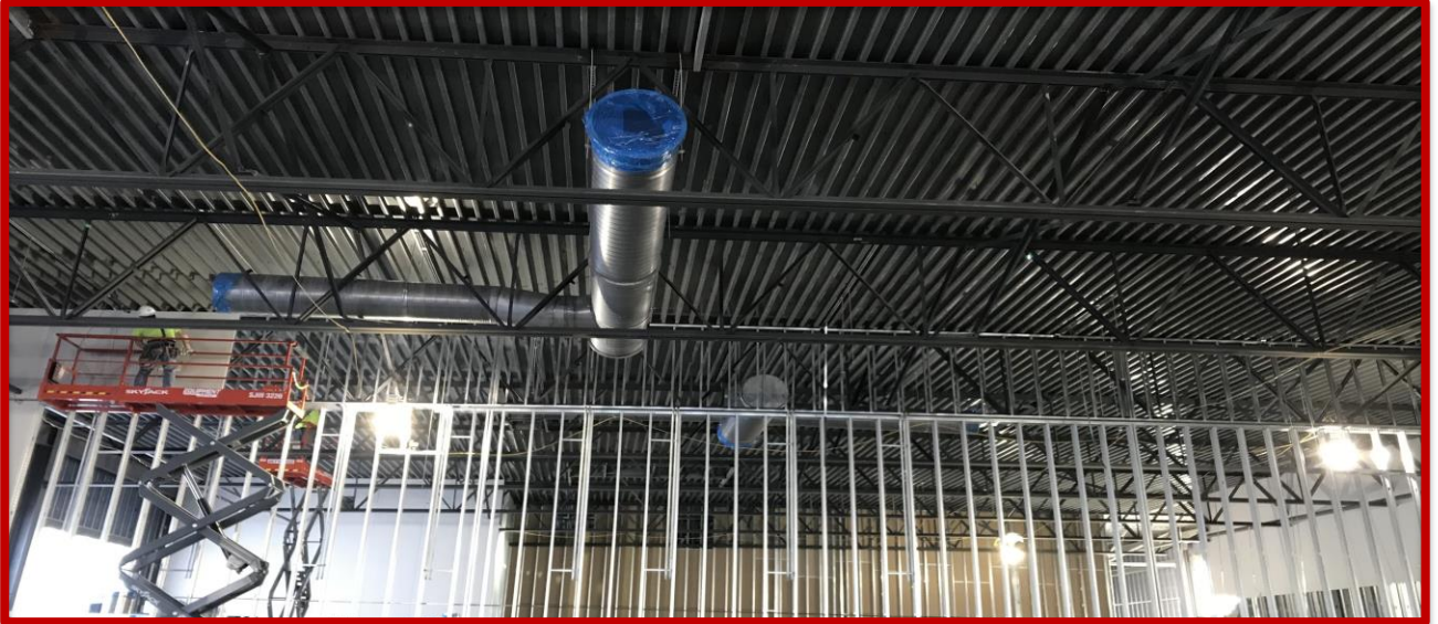
Picture 4: HVAC Ductwork in Area A
