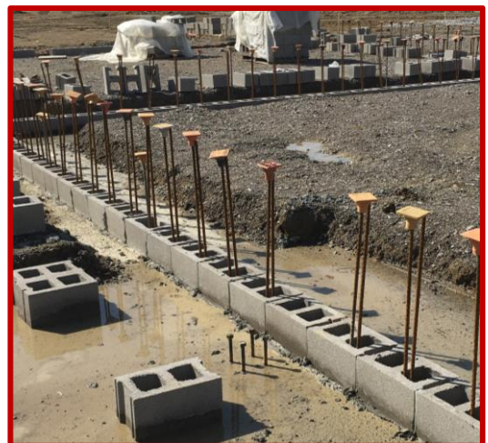
Picture 3: Progress on firewall masonry foundations
