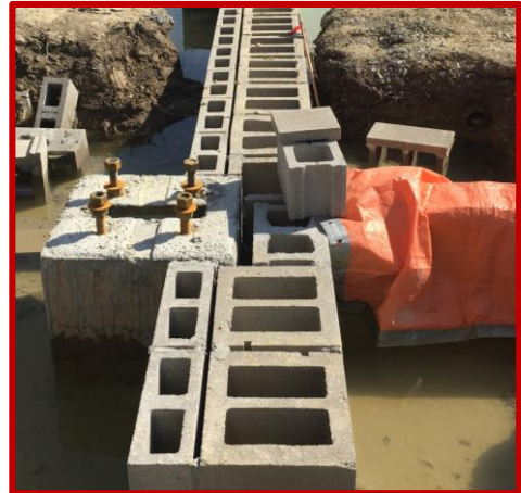
Picture 1: Masonry tie-in to concrete pier in Area D
