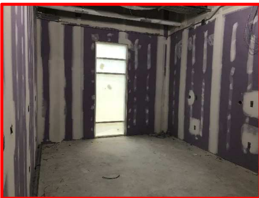
Picture 2: Finishing of Drywall in the Manicure Room
