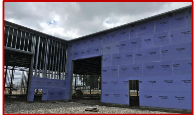
Picture 1: Progress of exterior sheathing in Areas A and C
