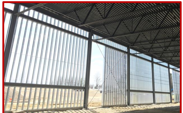
Picture 3: Progress of metal stud framing in Area A
