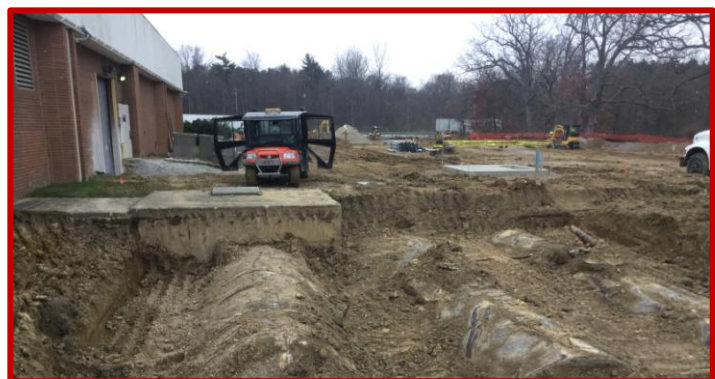
Picture 3: Exploration of storage tanks on north end
