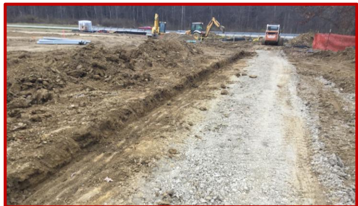
Picture 2: Progress on installation of gas line
