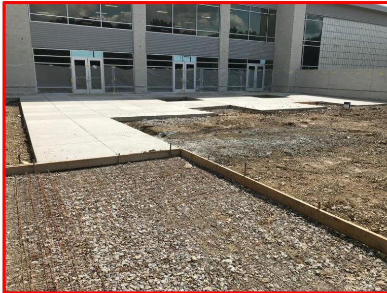
Picture 6: Concrete Progress on the West Side of the Building
