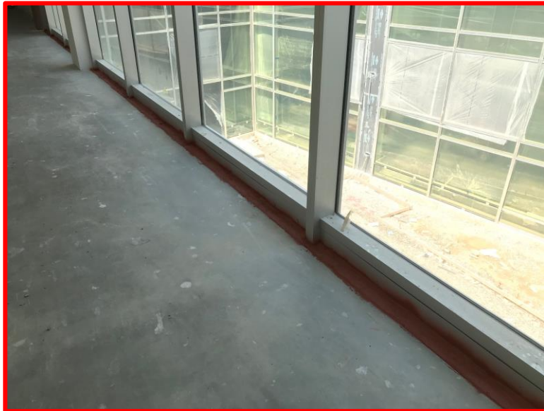
Picture 4: Fire Stopping on the Mezzanine
