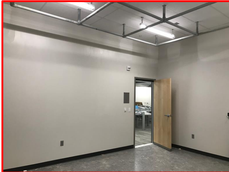
Picture 7: Progress in the Production Room
