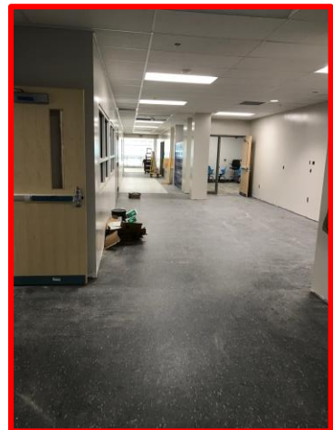
Picture 3: VCT in the Mezzanine Corridor
