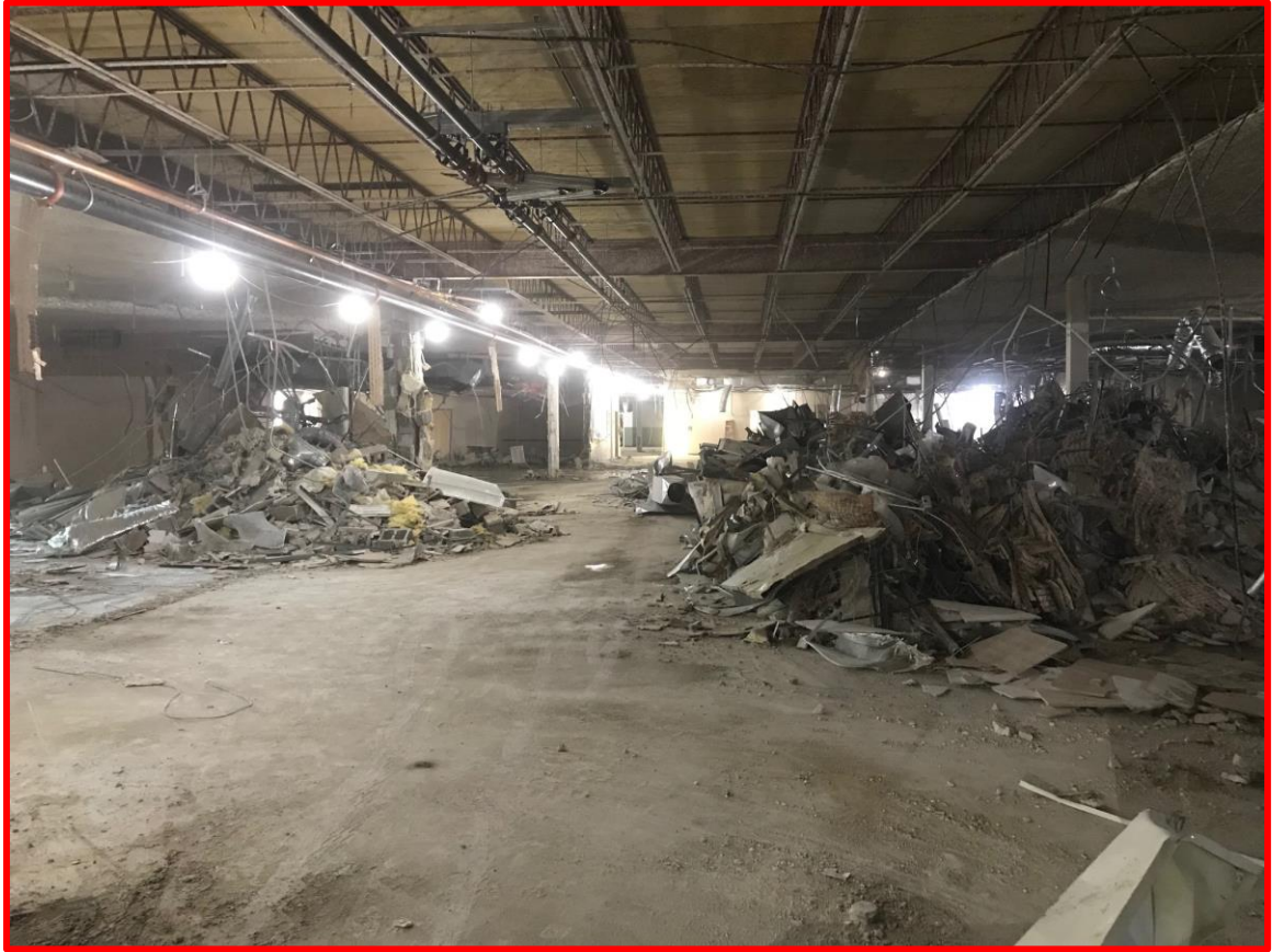
Picture 6: Selective Demolition Progress in the Existing Building
