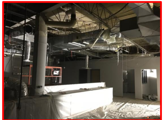
Picture 3: Selective Demolition in the Health Tech Area
