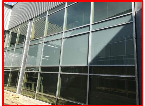
Picture 1: Spandrel Glass in the Connector Courtyard
