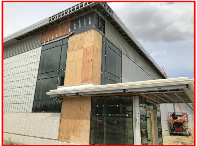
Picture 6: Southwest Entry Canopy and Glazing
