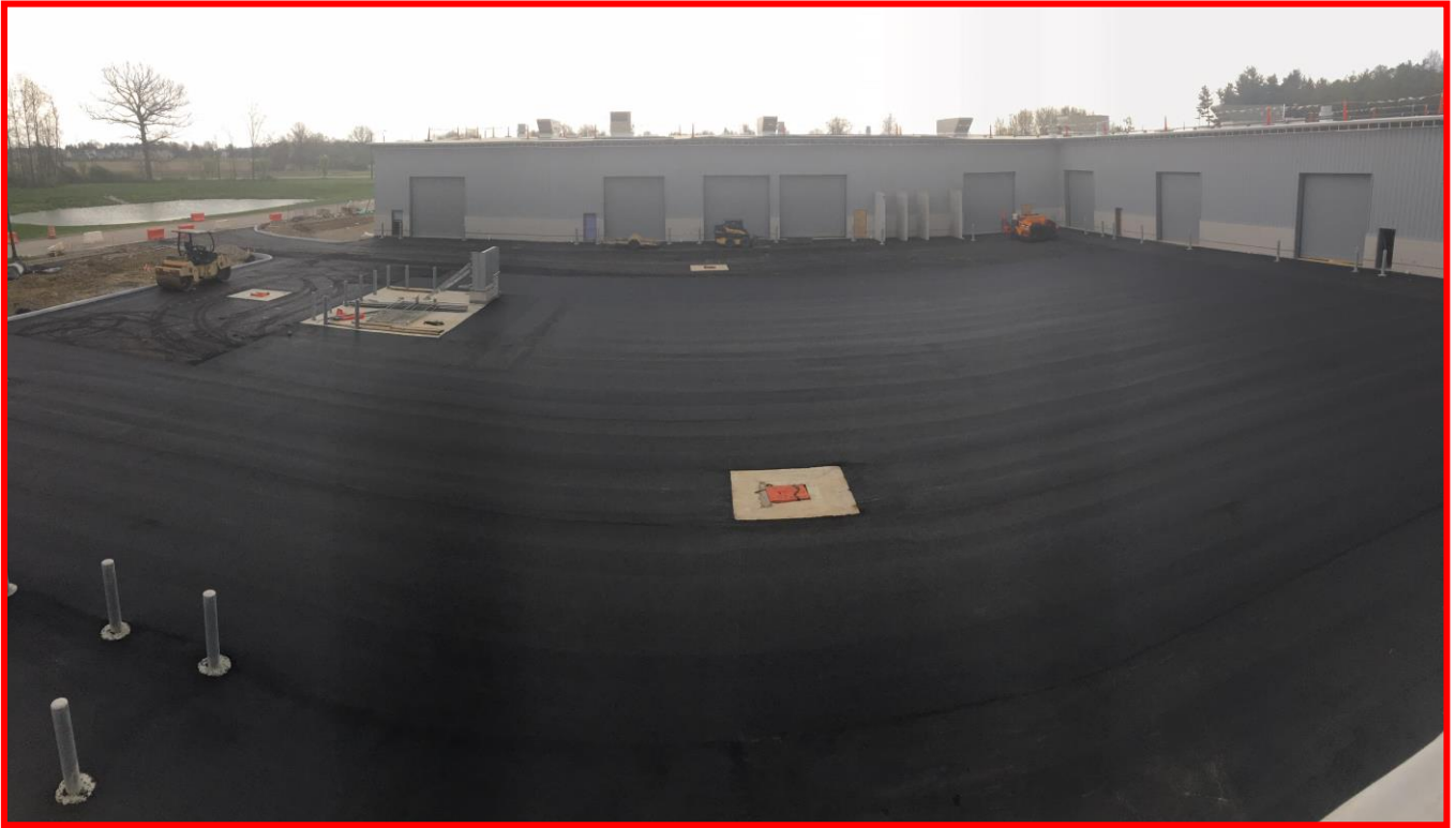
Picture 4: Asphalt Paving in Courtyard
