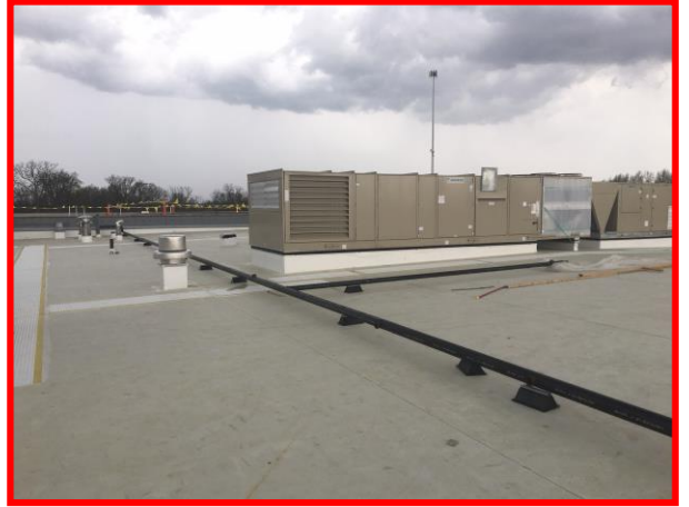
Pictures 7, 8: Main Gas Line on Roof
