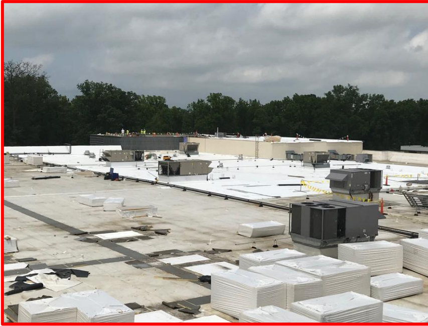
Picture 6: Progress of Re-roofing of Existing Building
