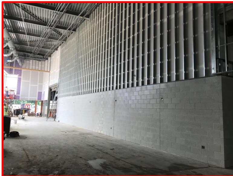
Picture 5: Masonry Veneer in the Connector
