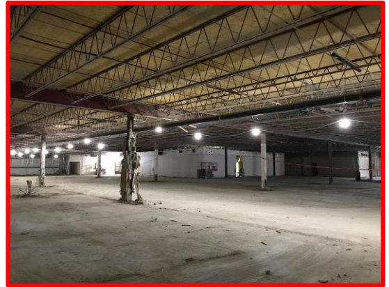
Picture 1: Selective Demolition Progress in the Existing School
