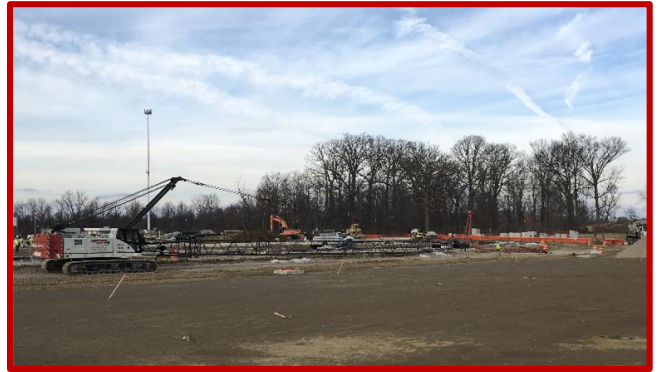
Picture 1: Finished assembly of the crane on-site
