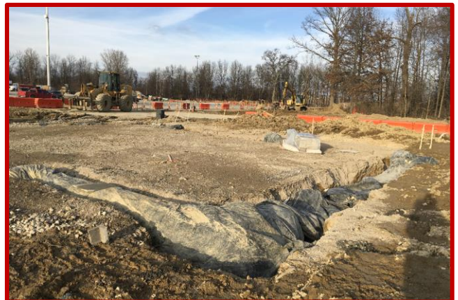
Picture 3: Protection of concrete foundation progress in Area E
