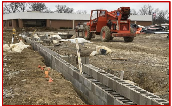
Picture 2: Progress on CMU foundation on the west side of campus
