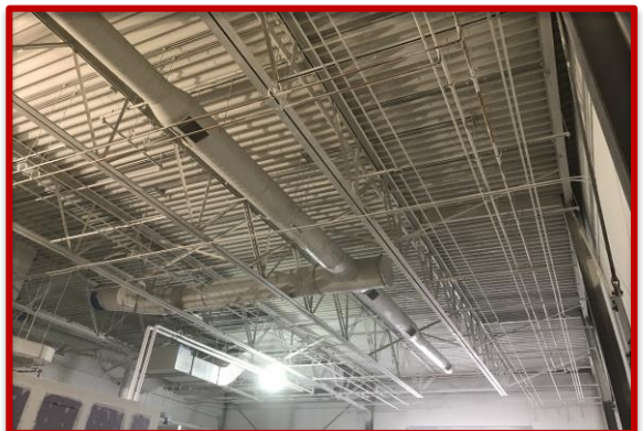
Picture 3: Painting Structure in Power Line Lab
