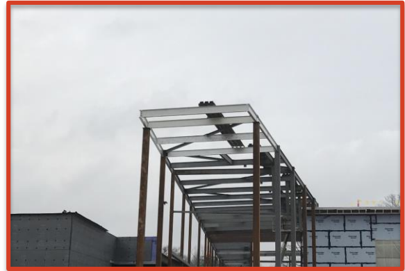
Picture 1: Signed Beams at Building Connector
