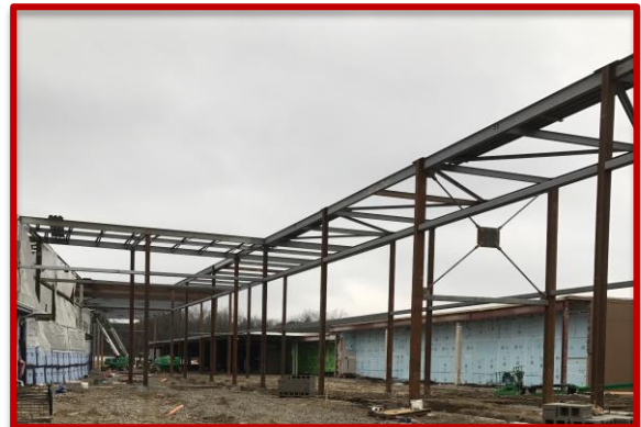
Picture 2: Steel Erection at Building Connector
