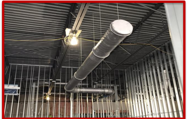
Picture 1: Ductwork Installation in Area B
