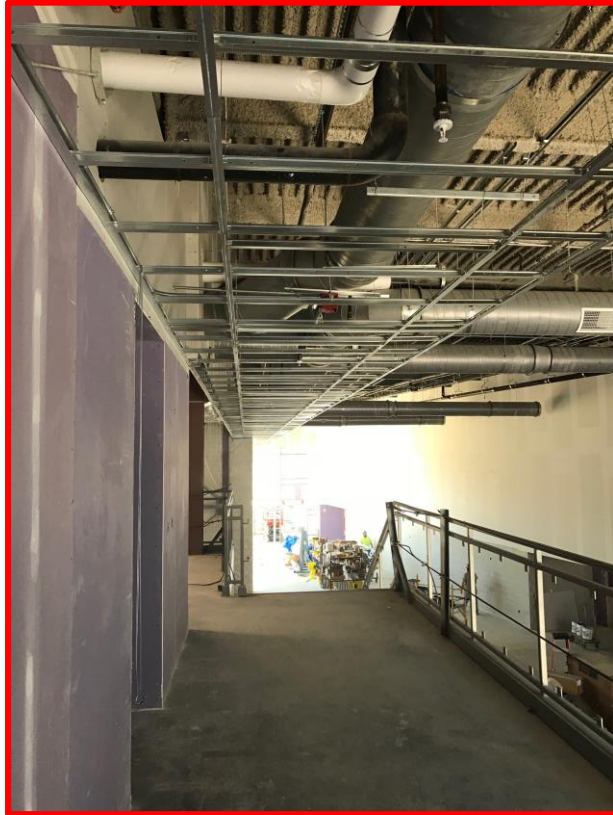
Picture 6: Suspended Gypsum Ceiling Installation on the 2 nd Floor
