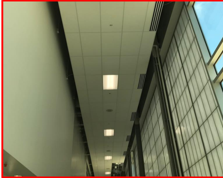
Picture 4: Ceiling Tile in the North-South High Bay Lab Corridor
