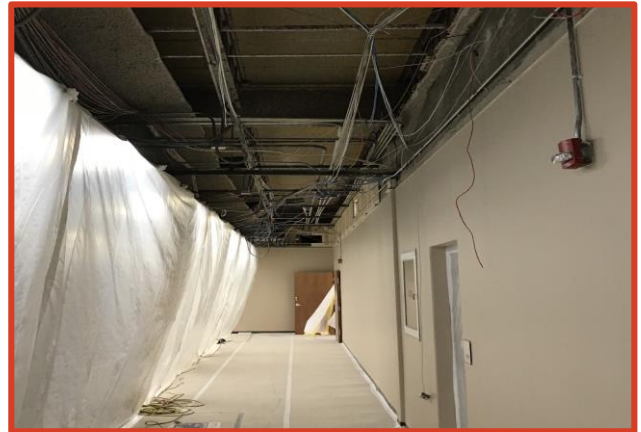
Picture 1: Existing Corridor for new Water and Fire Lines
