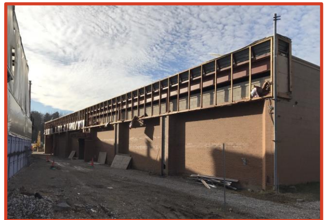
Picture 2: Transite Panels removed along South Elevation
