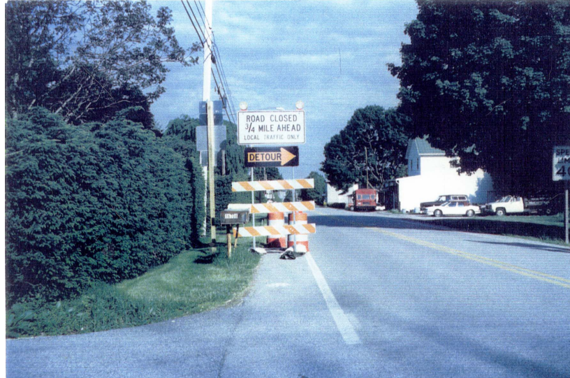
Figure 1. Type III Barricade Has Drums Behind It That Restrict Sight Distance
