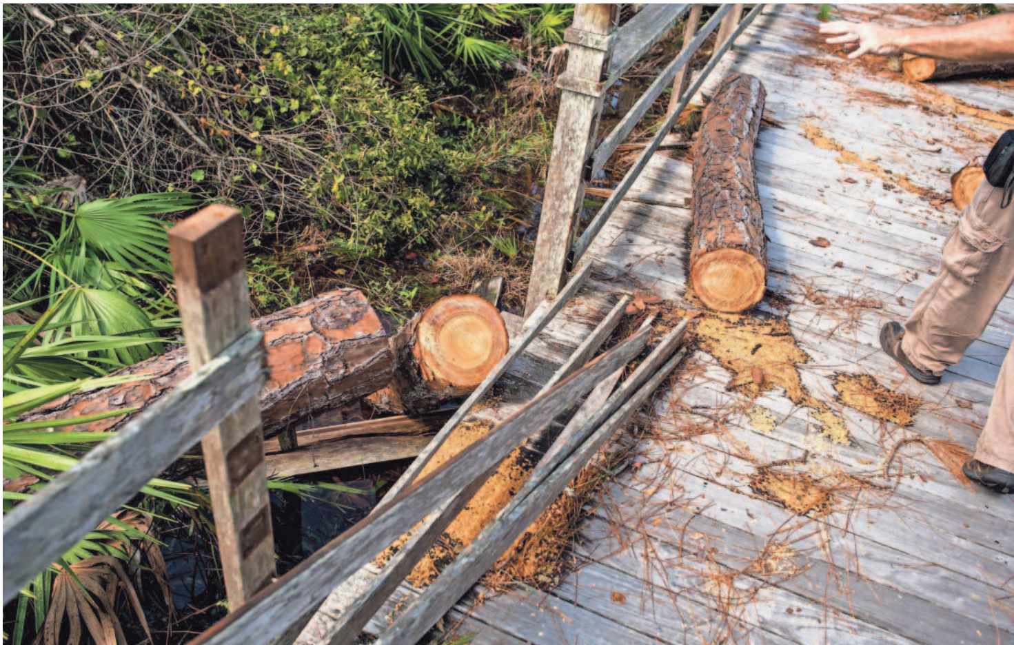
Handrails and side rails were damaged on numerous sections of the boardwalk in Corkscrew Swamp Sanctuary, but the boardwalk still is passable on some of those sections. JUSTIN GILLILAND/SPECIAL TO THE NAPLES DAILY NEWS
