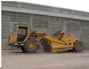
Excavation. Concrete Foundation
