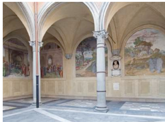
Cloister of the Vows, Basilica of the Santissima Annunziata, Florence, Italy (after restoration)
