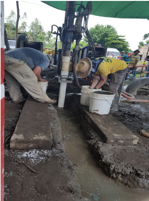
The team packs gravel around the casing.
