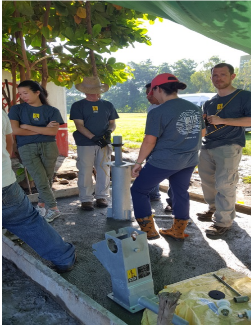
The team finishes added PVC piping and then installs the hand pump.
