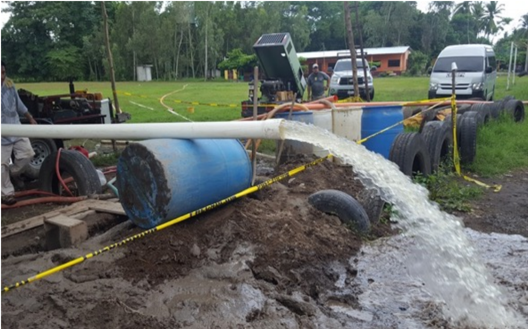
The team turns on the air compressor, and the first bit of water from the well flushes out. They continued flushing the well to ensure the borehole was free of debris.
