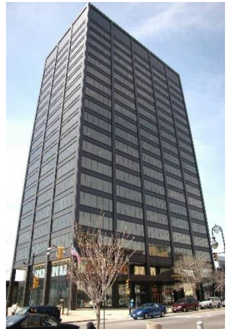
Below: The spectacular 24 Story Brady-Sullivan Tower in Manchester... the site of "LIVE UNITED Over the Edge 2018"
