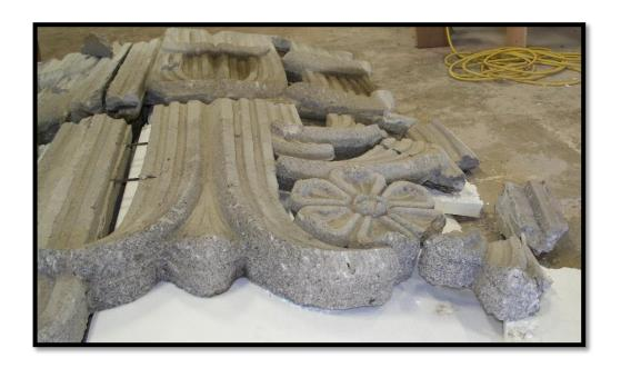
Unlimited Designs skilled craftsmen got right to work, reconstructing these panels, by filling in holes, re-sculpting missing details, and piecing back together parts, that time and weather had taken their toll on.
