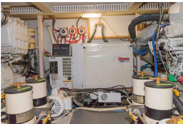
Onan Generator in Sound Shield Enclosure
