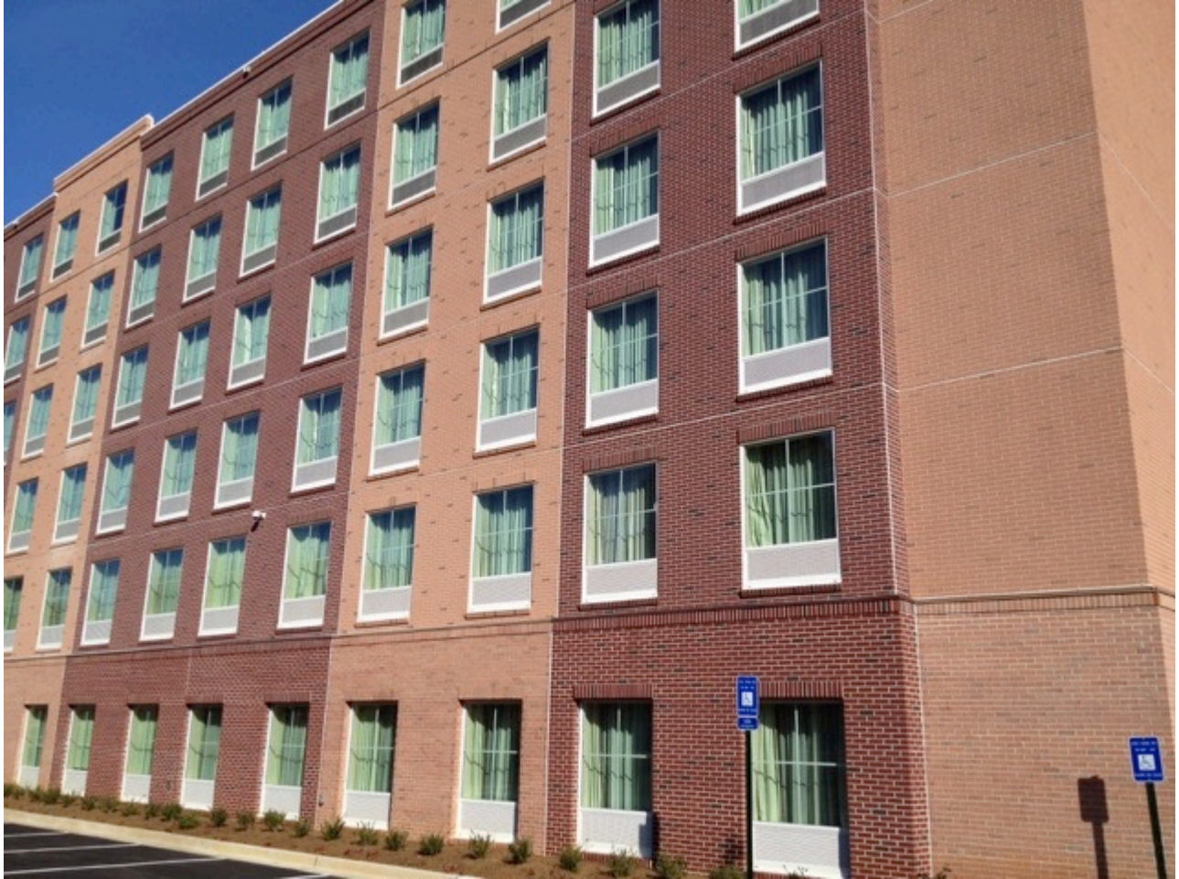
The Homewood suites in East Point, Georgia, made use of EIFS with a brick appearance on floors two through six that blended in with the first floor of clay brick and saved the project about $175,000 in material costs.
