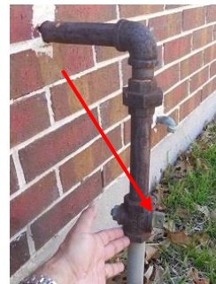
Gas riser valve open
