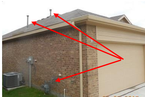
Gas flues on roof top and gas meter
