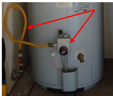
Yellow gas line and gas valve
