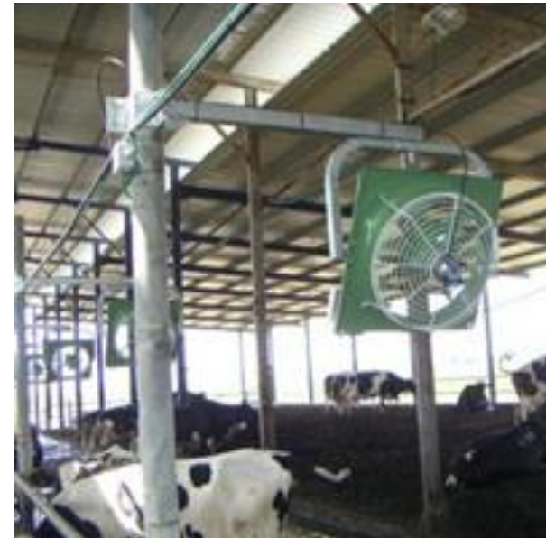
Monitor and/or control confinement buildings!
