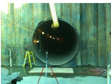
**Sandy River Conduit Relocation- OR.** Alcantar & Associates performed the survey construction staking for this project. Alcantar provided alignment for the 30-foot-diameter construction shaft to depth of 85 feet; two drilled 9-foot-diameter shafts to a depth of 110 feet and a 13 foot-diameter modified horseshoe tunnel running diagonally under the girder of the Sandy River. Alcantar & Associates provided marking coordination, differential leveling and monitoring as well.
