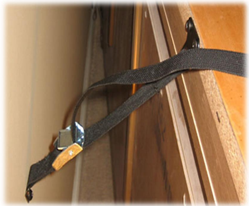
Dresser secured to the wall
