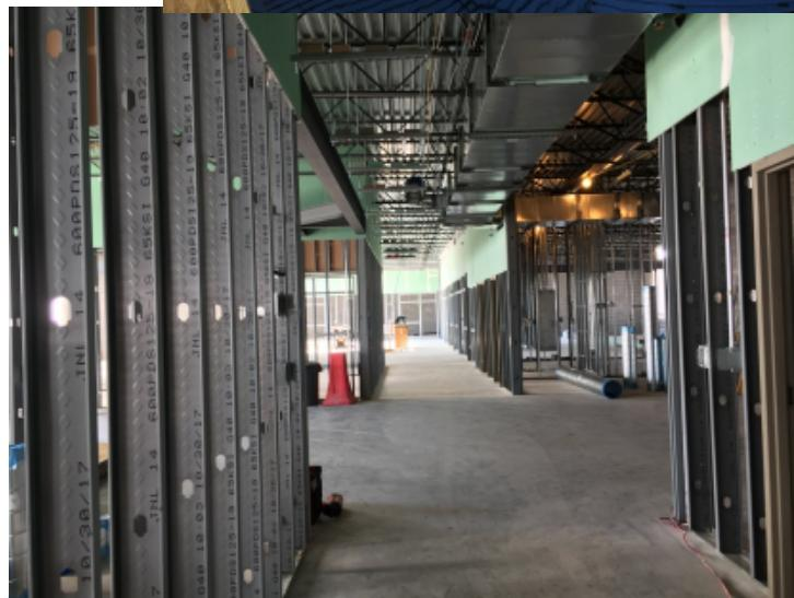
Roofing for the classroom wing is near completion and will finish next week. Metal decking for the courtyard has finished. Drywall framing for the Upper Level is complete.
