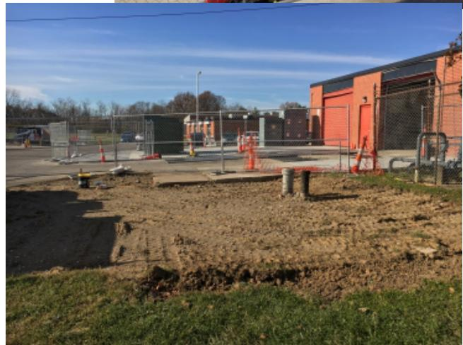
**Electrical work has finished and the shed has been demolished. Slab preparation has started for the new dumpster pad.**
